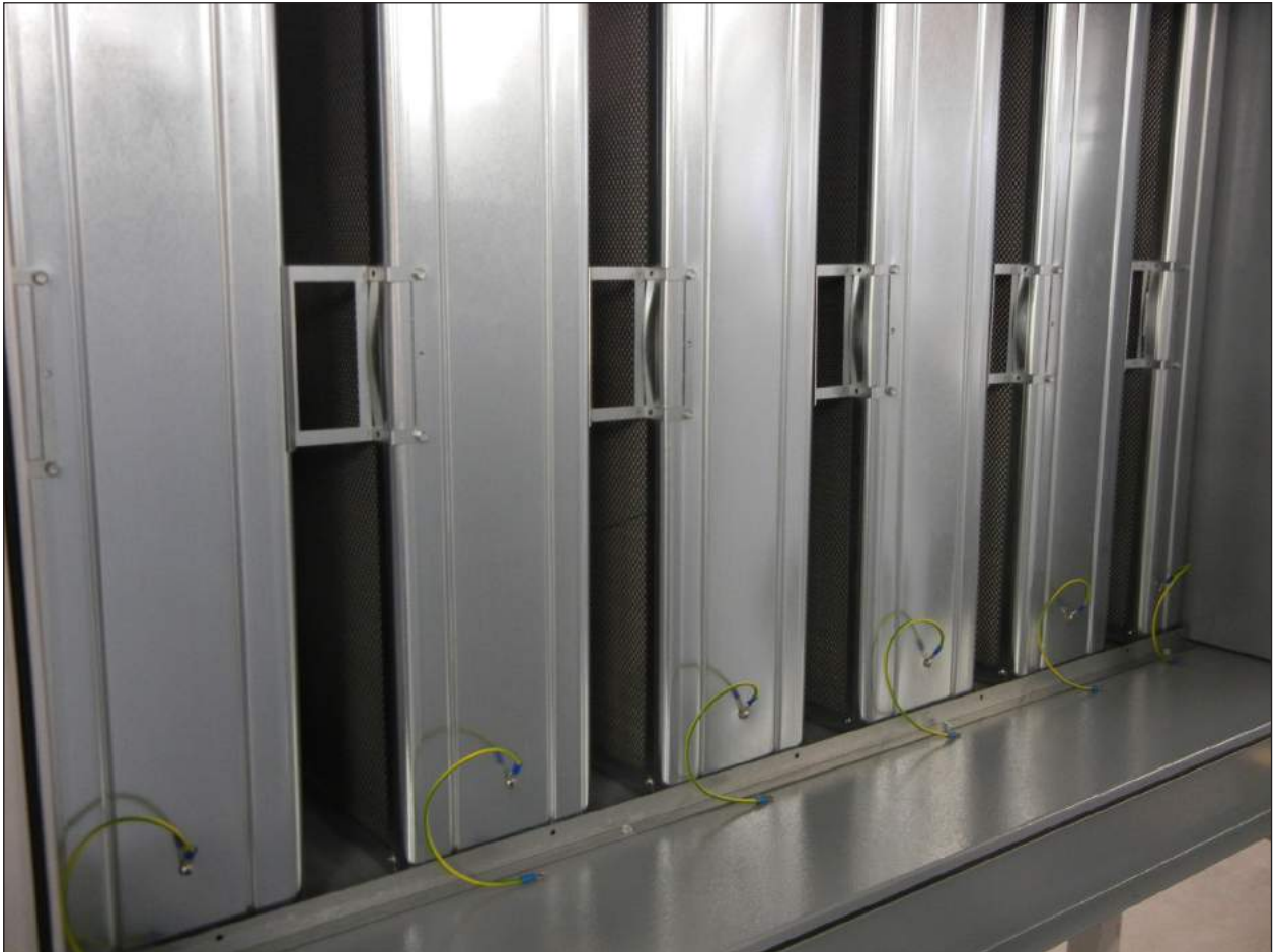
Fig. 66 Multiple silencer baffles with equipotential bonding
