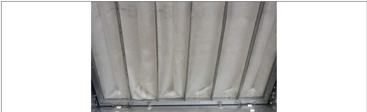
Fig. 79 Filter mounting frame with filter clamps
