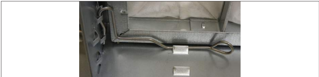
Fig. 77 Filter mounting frame, left filter clamp
