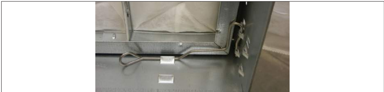
Fig. 78 Filter mounting frame, right filter clamp
