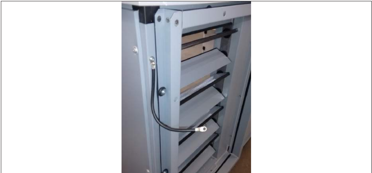
Fig. 16 Potential equalisation mounted on the unit
