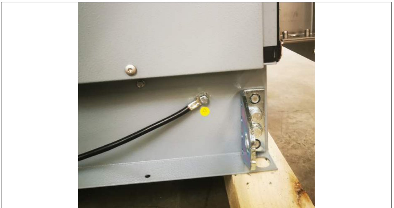
Fig. 15 Potential connection on the base frame
