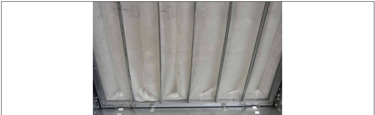
Fig. 79 Filter mounting frame with filter clamps
