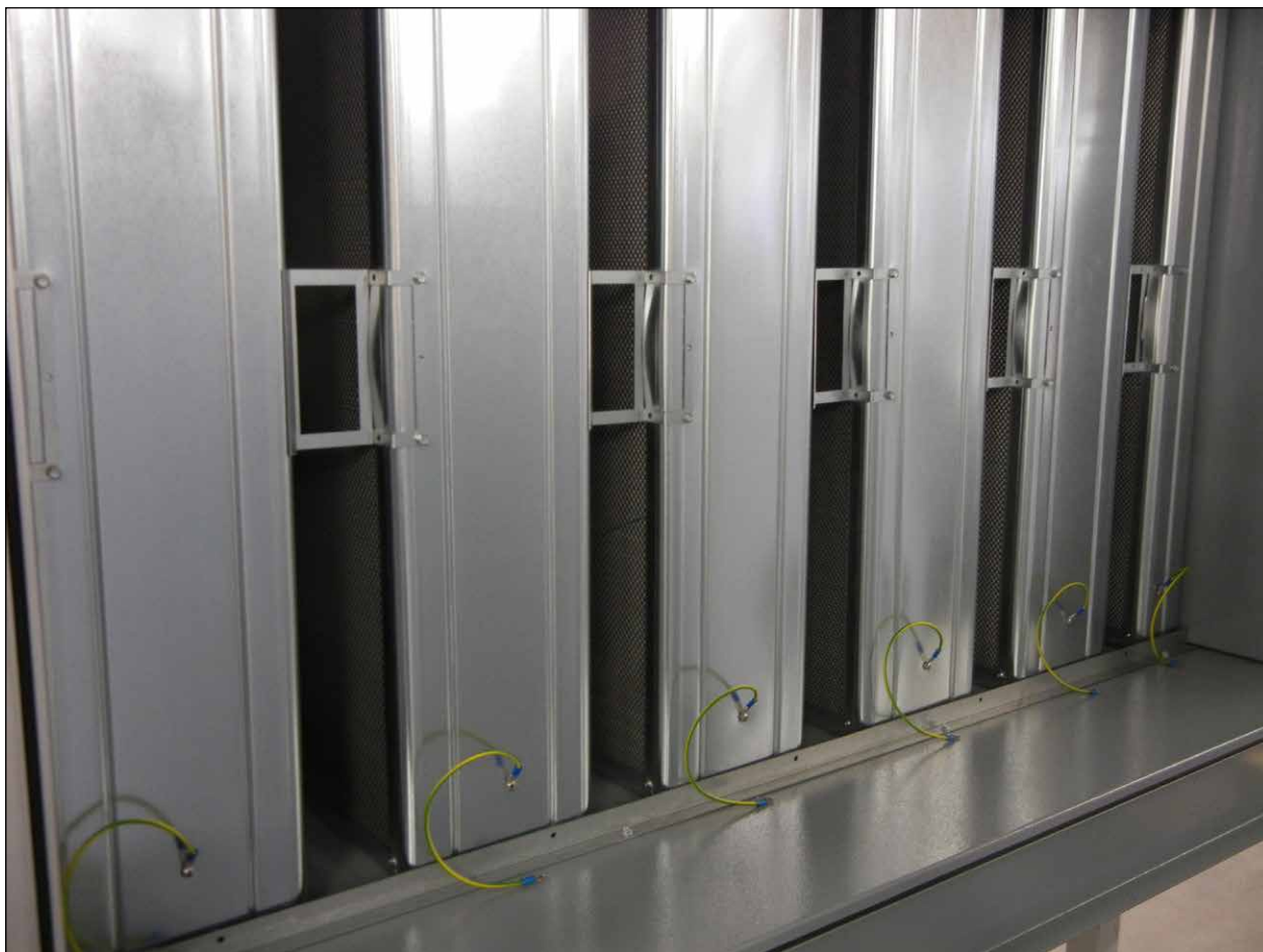
Fig. 66 Multiple silencer baffles with equipotential bonding
