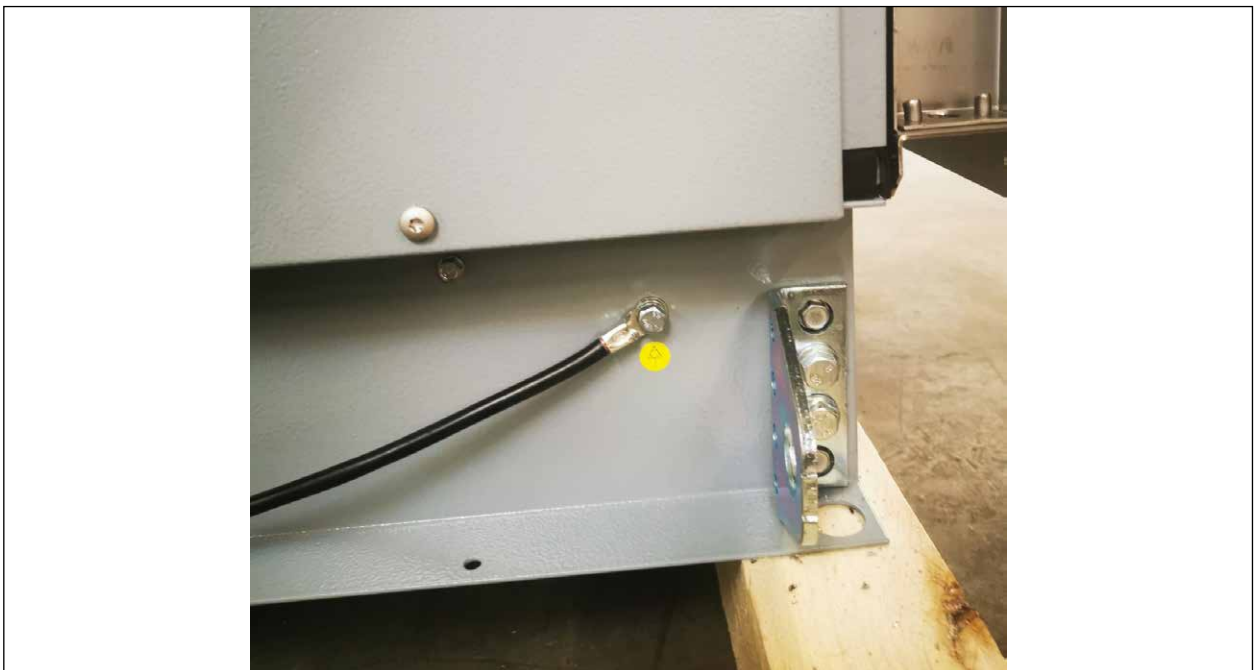
Fig. 15 Potential connection on the base frame
