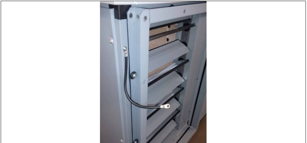
Fig. 16 Potential equalisation mounted on the unit
