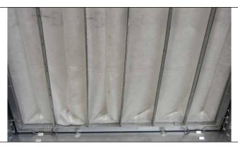
Fig. 70 Filter mounting frame with filter clamps
