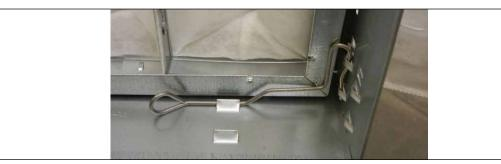
Fig. 69 Filter mounting frame, right filter clamp
