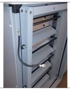
Fig. 6 Potential equalisation mounted on the unit
