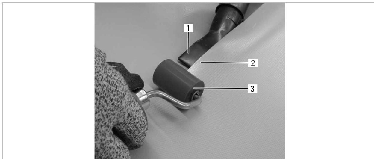
Fig. 29 Sealing of the roof membrane via hot air welding
