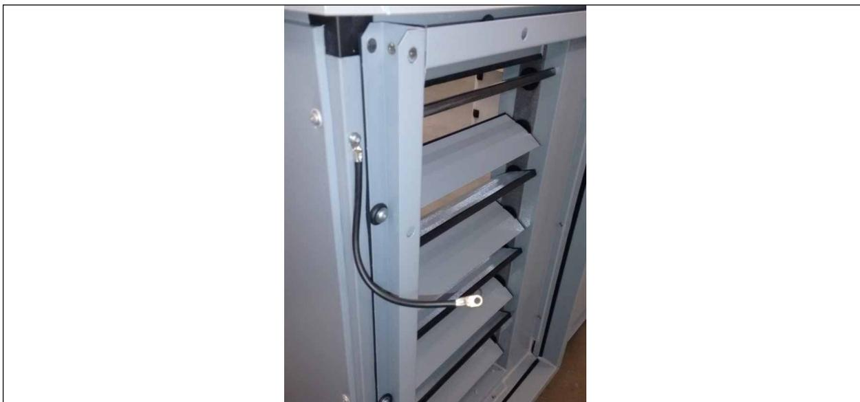
Fig. 6 Potential equalisation mounted on the unit
