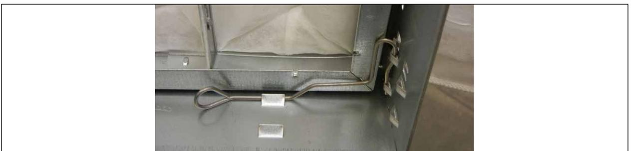
Fig. 69 Filter mounting frame, right filter clamp
